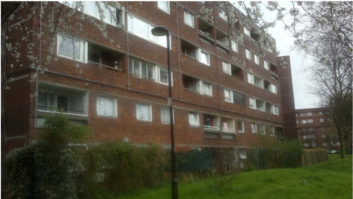
Photograph 1-showing Rhodeswell Road Block
